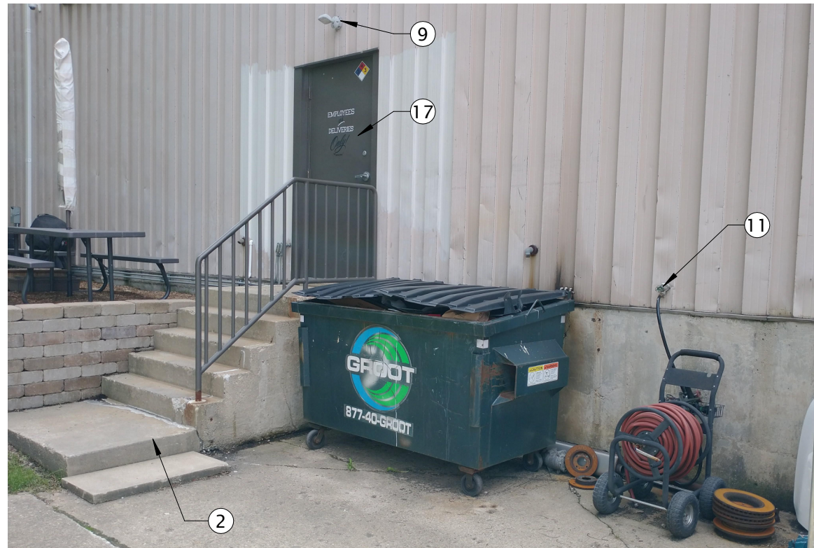
EXISTING BUILDING – REAR ENTRY
