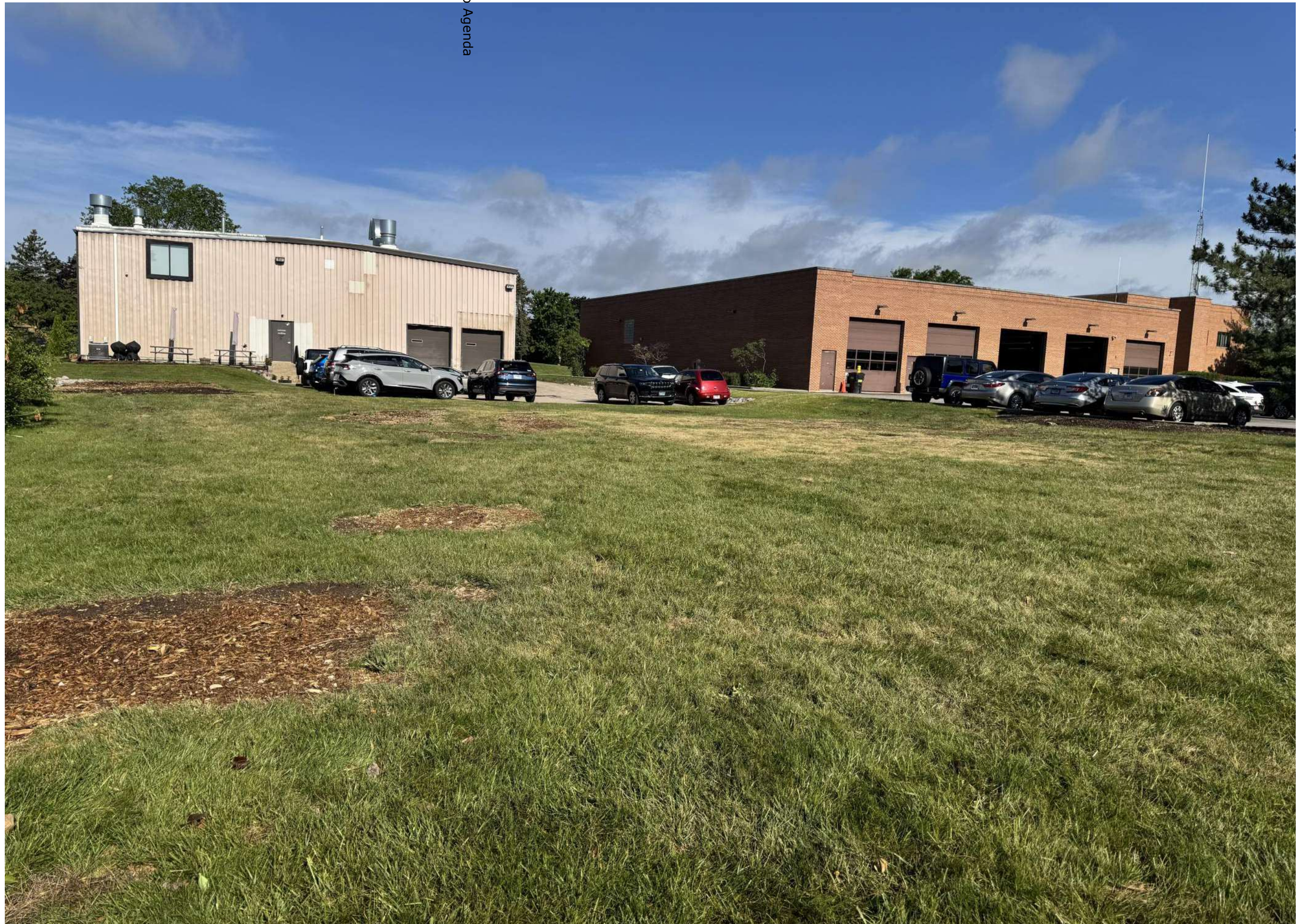
121 Schelter Rd Parking Lot Current rear yard
