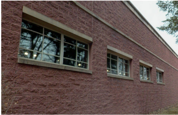
Existing rear / east-facing wall with high-set windows.
