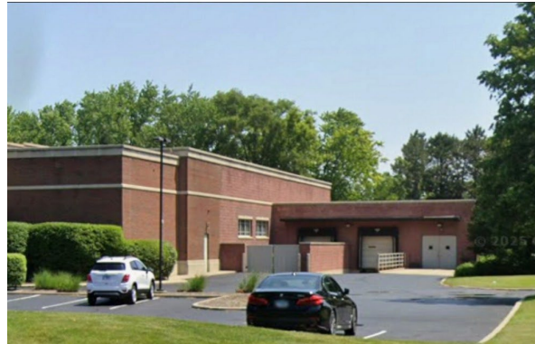
Existing east service area and loading doors.
