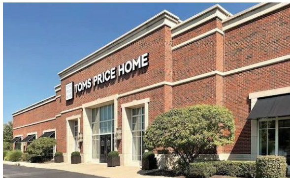
Existing front entrance and primary façade.
